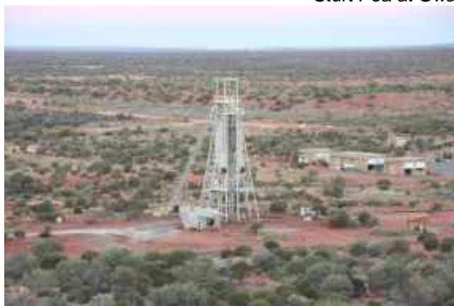
Headframe at Mt Windara Nickel project Viewed from Mount Windara lookout
