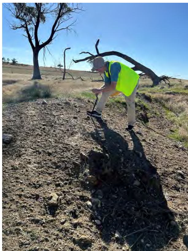
James inspecting a trench.
